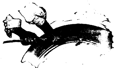
Fig. 14. Placing Tire on Rim, Third Position.
