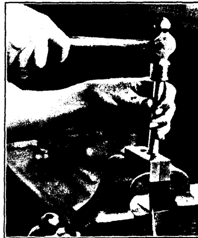
Fig. 21.—Pipe Flanging Tool 71974
