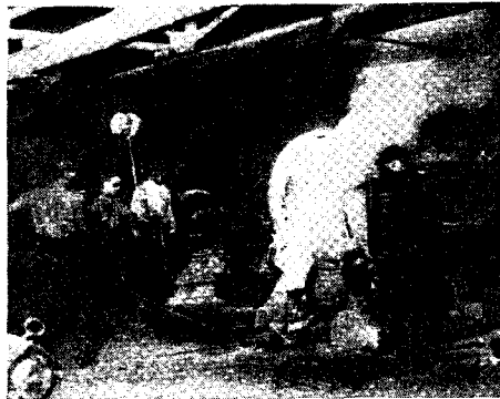
All bronze bushings and brass parts are cast in Cadillac-La Salle foundries. The metal is melted in electric furnaces, then is poured into ladles from which it is repoured into sand moulds
