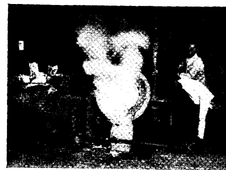
Pouring aluminum. The white-hot silvery metal is poured into sand moulds to form LaSalle parts
