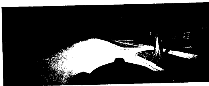
Fig. 15a. The "City Driving" position amply illuminates the street for driving where there is little or no traffic.
