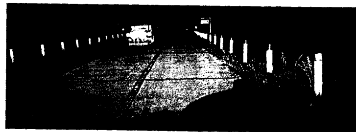
Fig. 23. Conventional Upper Beam aimed high enough to provide safe road lighting on rolling and winding roads.
