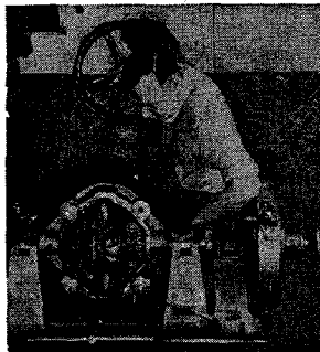
Matching Rear Axle Gears in a "Quiet Room" Test
