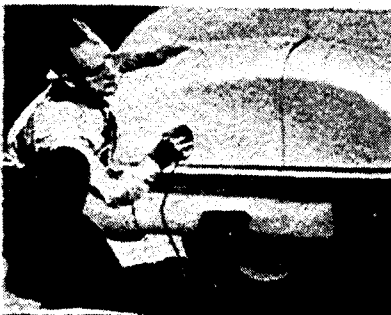
CHECKING LACQUER THICKNESS
