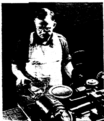
BEARINGIZING WRIST PIN HOLE
